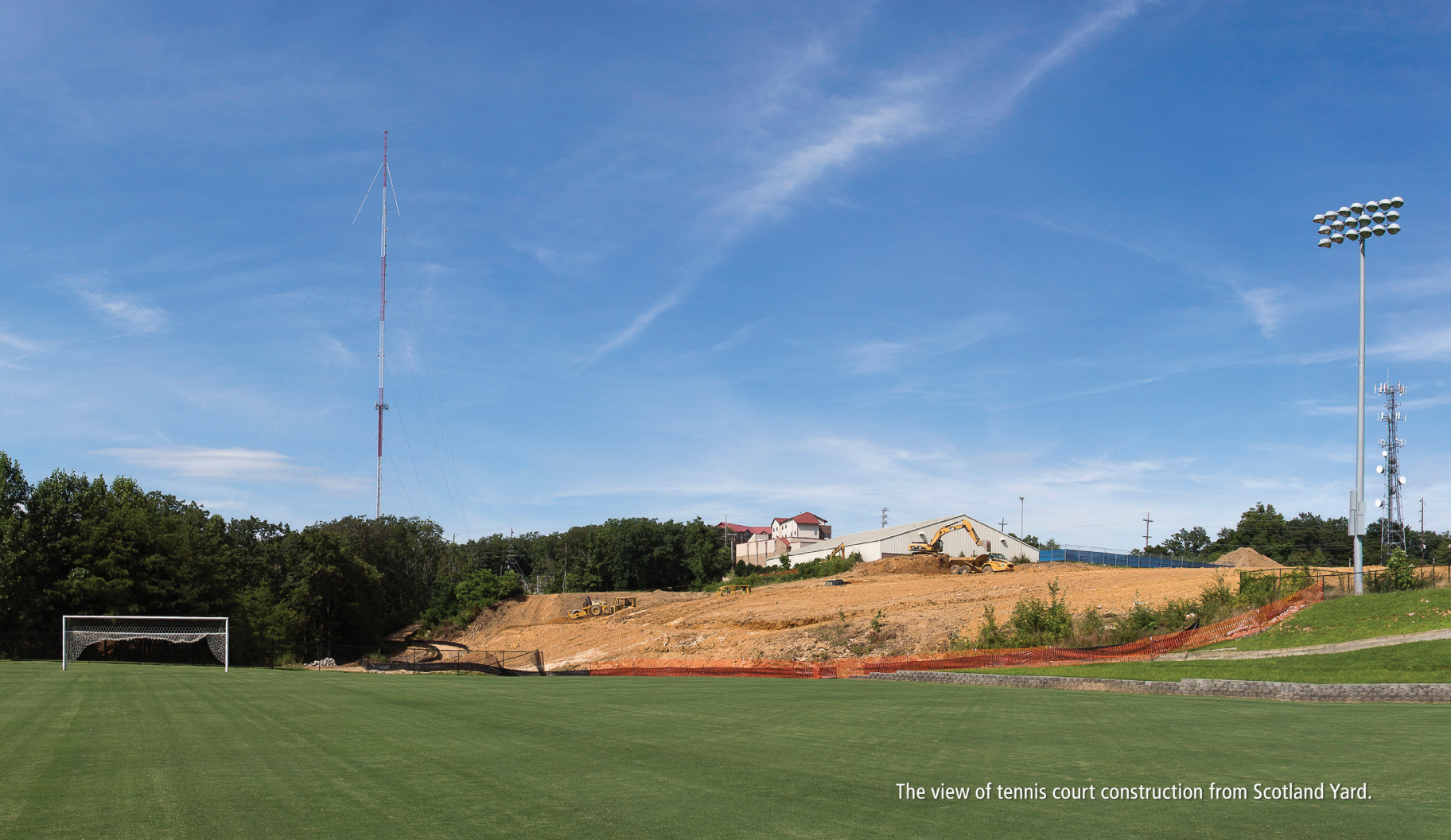
Construction teams lay the foundation for six new tennis courts.
